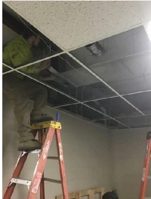
Ceiling Grid and Tile Being Installed in Hallway
