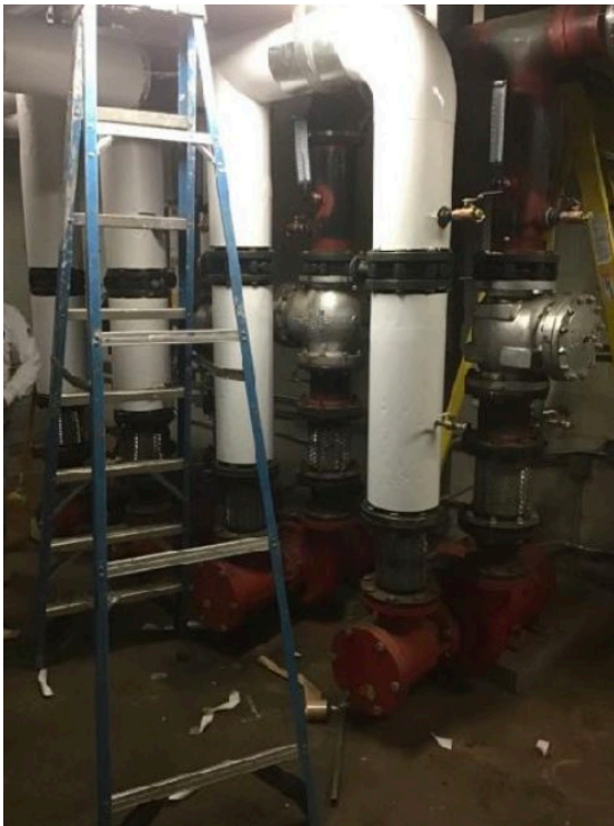
Insulation of Pipes in the Boiler Room
