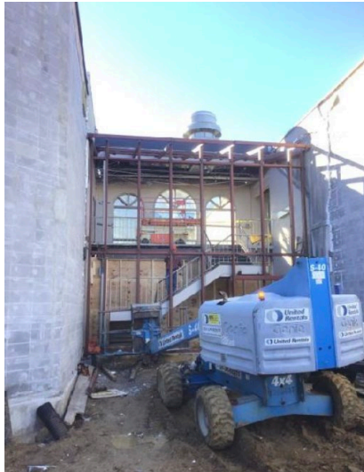
Steel Work Connecting Buildings
