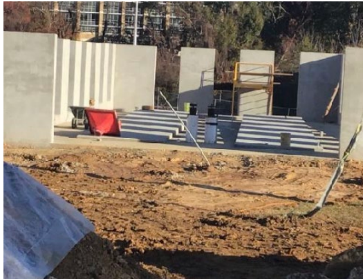
Concrete Pad for Chiller Installation
