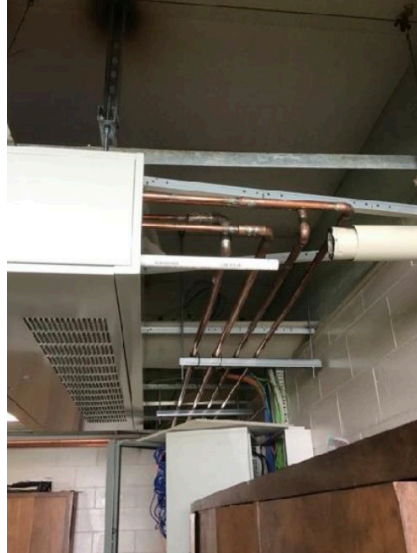
Piping Connected to Fan Coil Units
