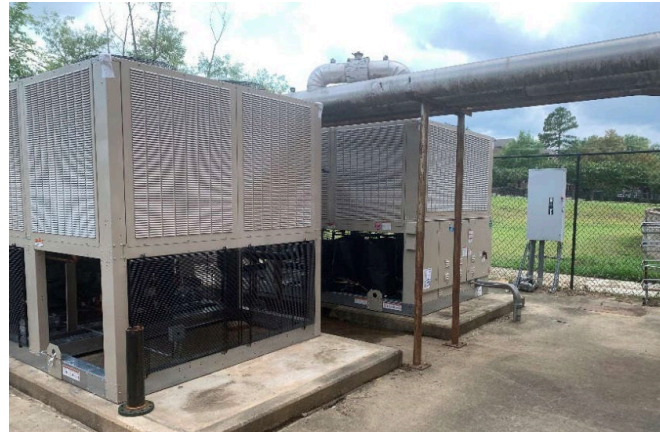
Chiller Installed and Operational (McWillie Elementary School)
