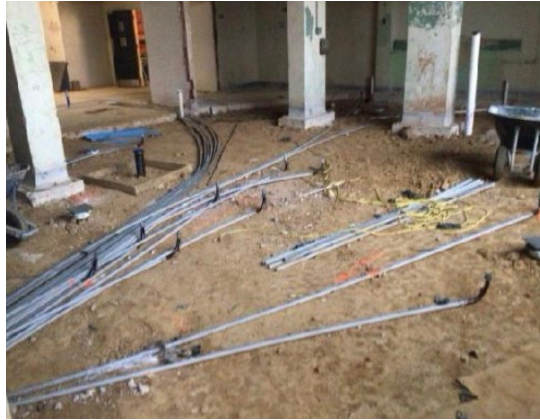
New Electrical Conduit Installed in the Kitchen
